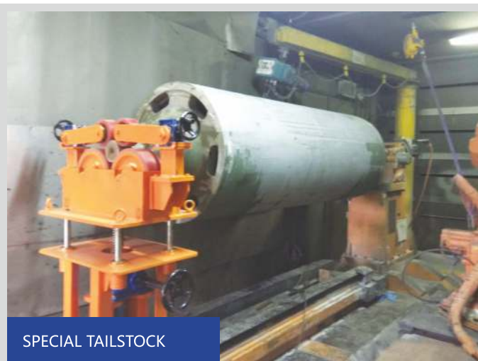
S S TANK WELDING SYSTEM
